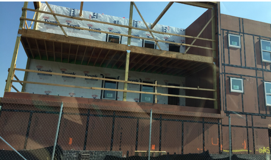
Centerville Neighborhood Branches at Centerville Housing Under Construction (Summer 2017)
