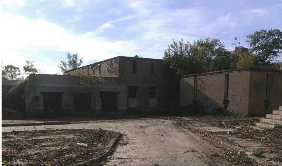
Catalyst Site - Camden Labs Prior to Assessment and Remediation, Fall 2016
