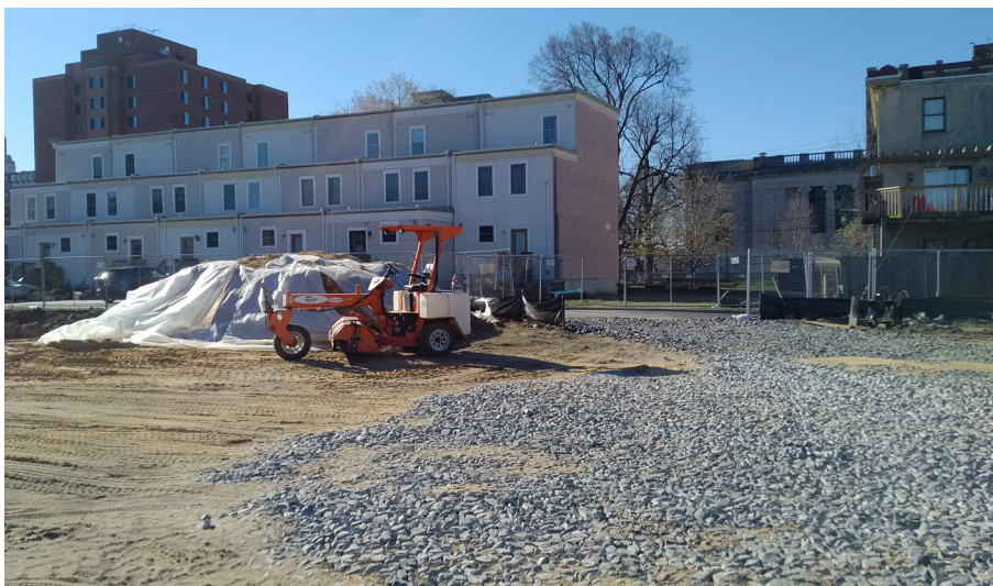
Site Remediation in Progress ABC Barrel Site, Camden, New Jersey
