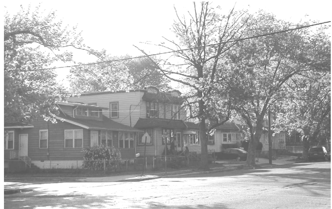
Typical Rosedale Single-Family Houses: 34 th & High Street
