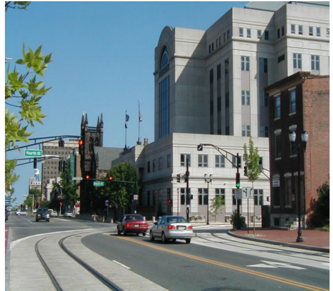
COOPER STREET: FEDERAL COURTHOUSE
