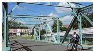
State St Bridge Improvements - Camden County • 2013 • $11.9 Million
