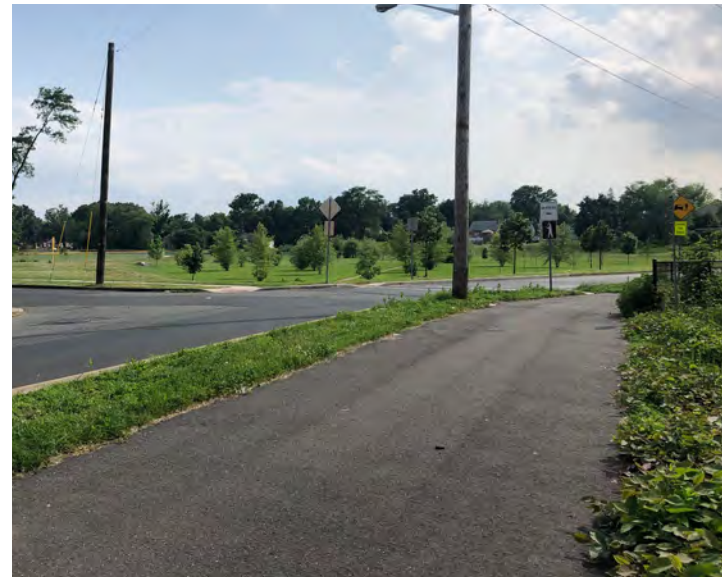
Baldwin's Run daylighting project along with several other green infrastructure initiatives have helped minimize the impact of flooding
