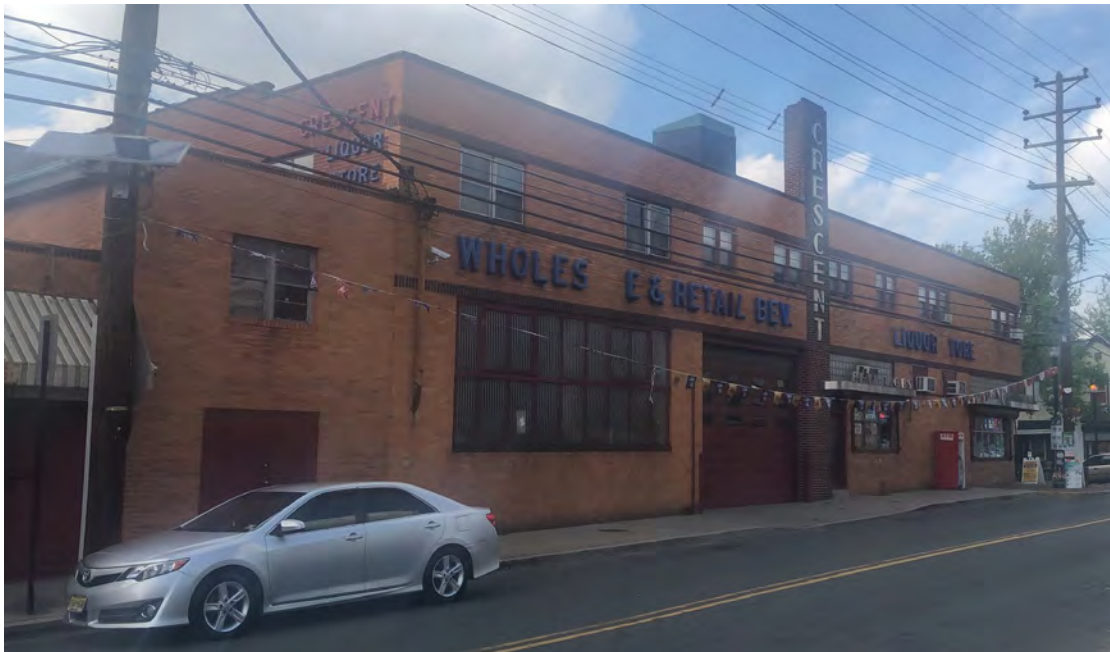
Crescent Beverage, located in an iconic building on the corner of River Ave and 25th St has been in business at that location since 1937.
