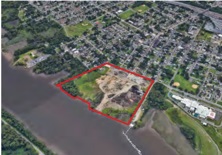
Riverfront Recycling and Express Marine remains as a legacy industrial use along the waterfront
