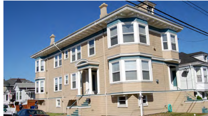
Example of small multifamily apartment building
