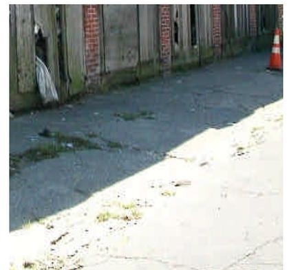
Image 21. The sidewalk conditions shown above present a safety hazard to pedestrians, the elderly, wheelchairs and strollers.
