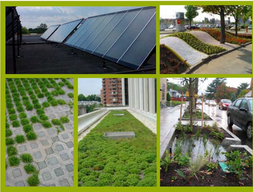
Green building and stormwater management techniques and materials: solar panels, planted berm, permeable pavers, green roof, infiltration bed.
