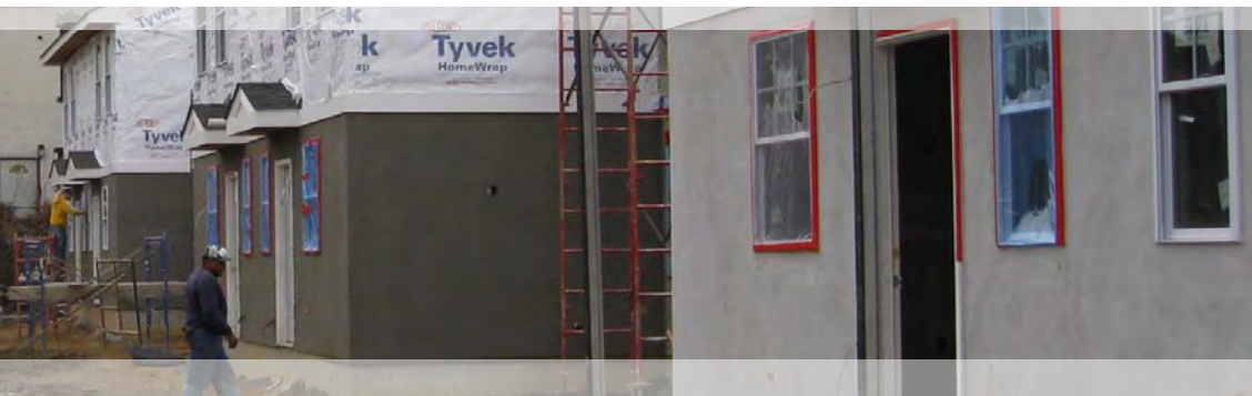
Construction underway at Camden Lutheran Housing's Grace II. Source: SOW
