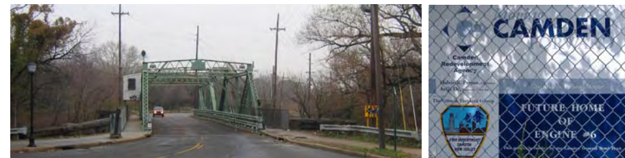
Sites of new State Street Bridge and Fire House.
