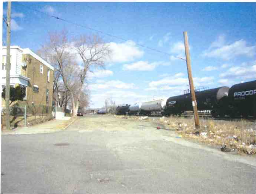
View of the rail line along Cleveland Avenue
