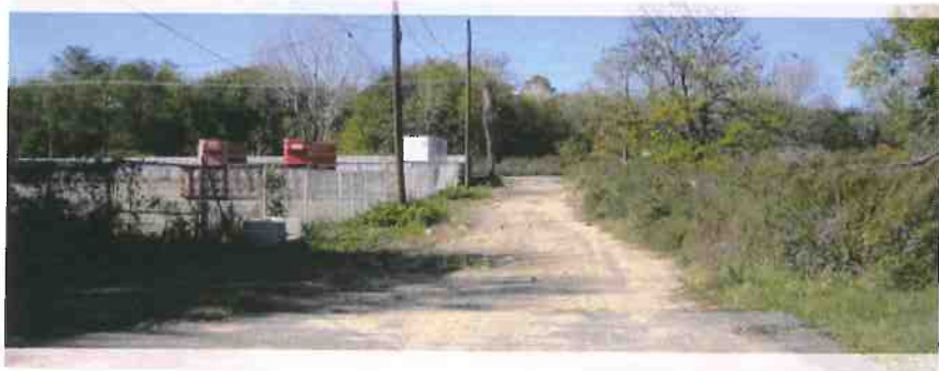
Poor street conditions are the product of poor maintenance and intensive truck use. In some cases, streets are just dirt roads in need of basic upgrades.
