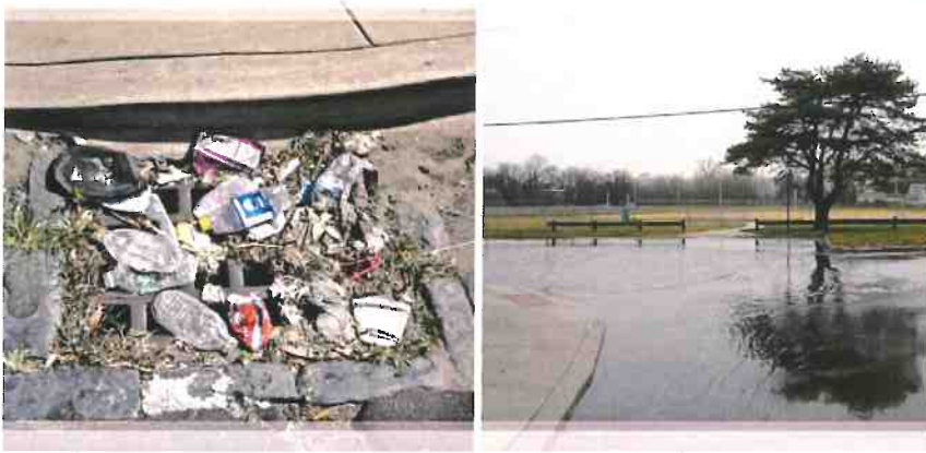
Even light rains can cause flood conditions at Von Neida Park. Cramer Hill's pervasive litter exacerbates street flooding by clogging storm drains and sewer inlets.
