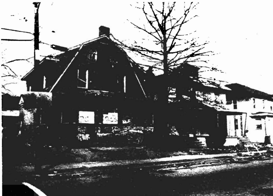
Housing abandonment, vandalism and even arson are not strangers to Stockton. Fortunately, the incidence of property vacancy is the lowest in East Camden.
