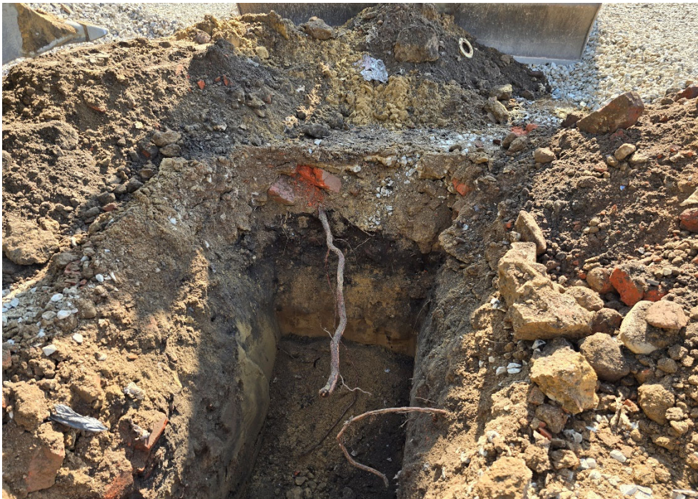
September 12, 2024 – Test pit TP-2
