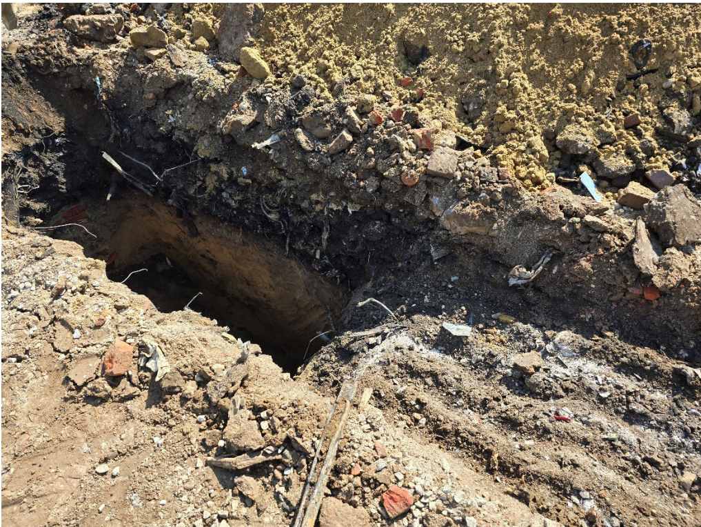
September 12, 2024 – Test pit TP-8
