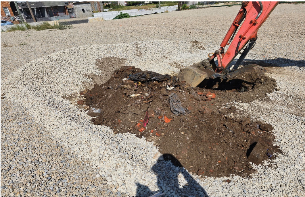
September 12, 2024 – Test pit TP-12
