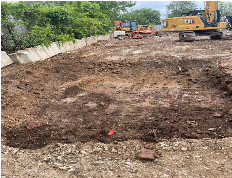
May 13, 2024 – Excavation of AOC-9b completed down to two feet below grade.
