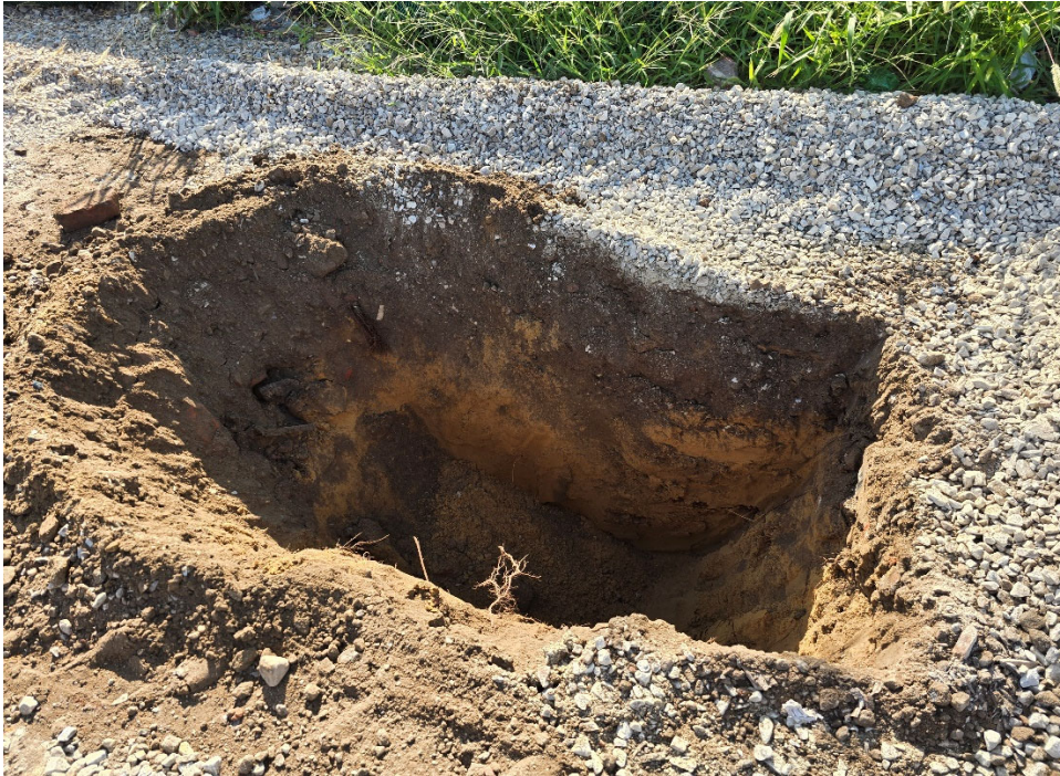
September 12, 2024 – Test pit TP-1 near MW-1.
