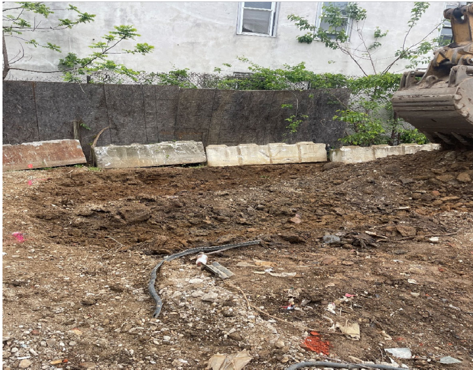
May 13, 2024 – Historic fill (brick and debris) observed within excavation of AOC-9b.
