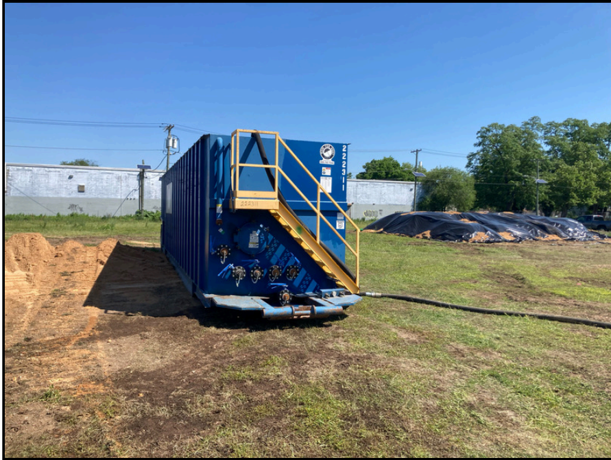
Frac tank used to store residual water and product mixture removed from USTs
