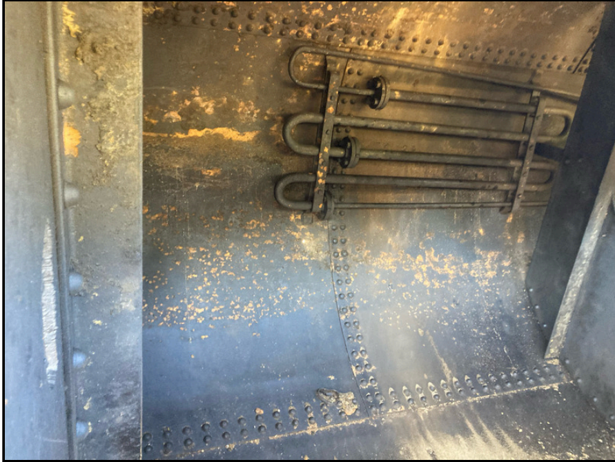
Interior of AOC 1E; heating pipes are pictured
