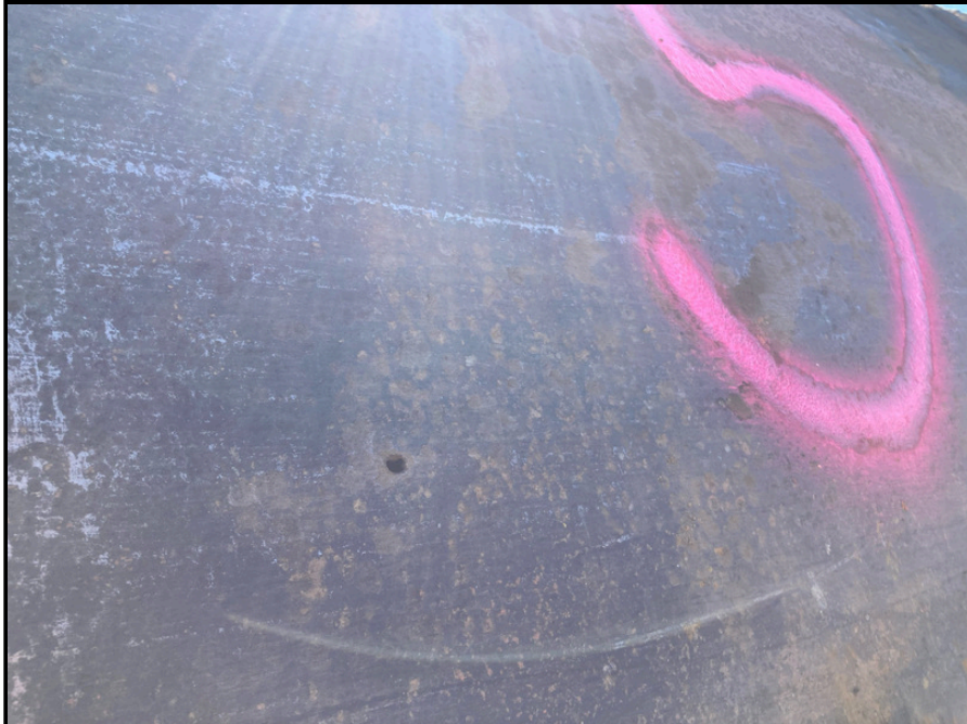
Holes in the bottom of AOC 1D
