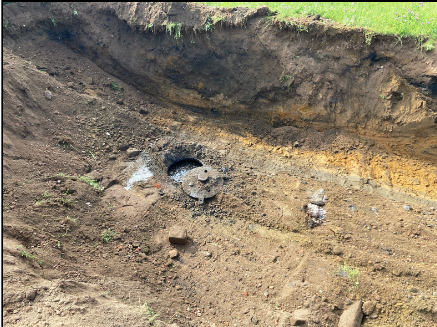
Exposed top of AOC 1A; residual water and product is visible within the UST
