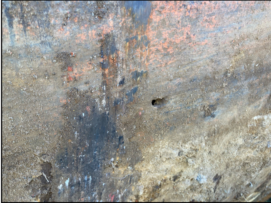
Holes in the bottom of AOC 1D
