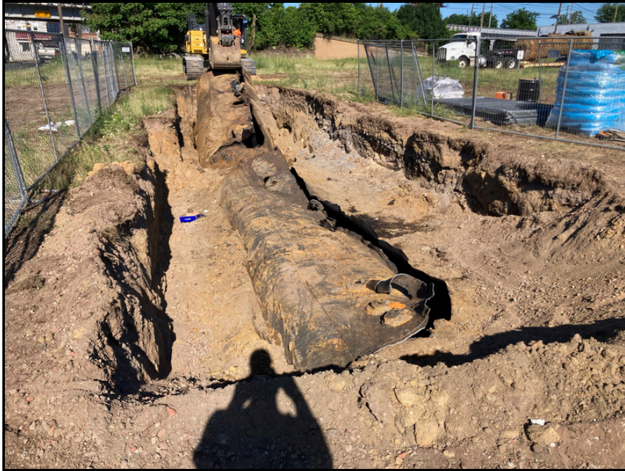
Exposed tops of AOCs 1D and 1E; AOC 1E is being removed
