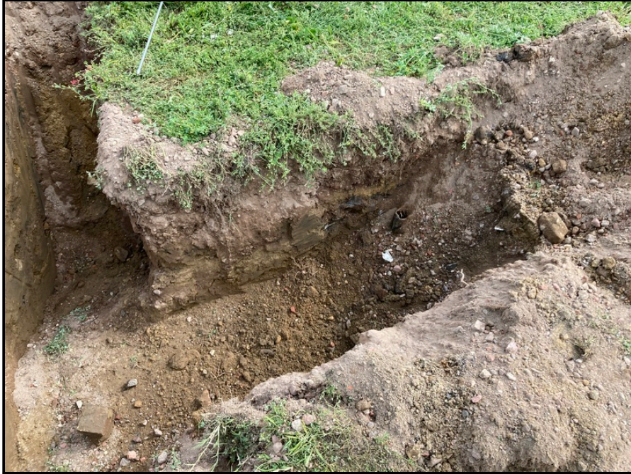
Excavation daylighting AOC E; fill port is visible
