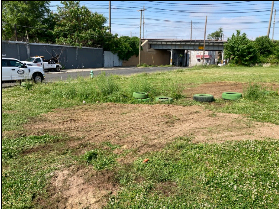
Backfilled excavations of AOCs D and E
