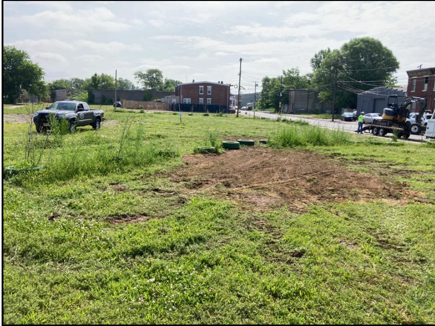
Backfilled excavations of AOCs D and E
