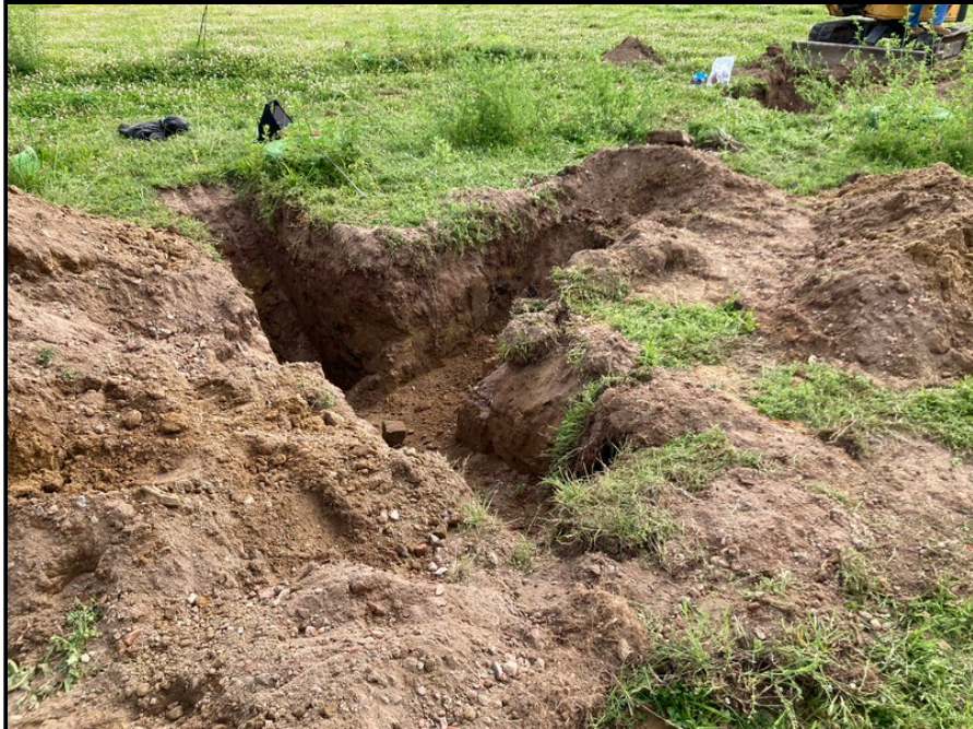
Excavation daylighting AOC E
