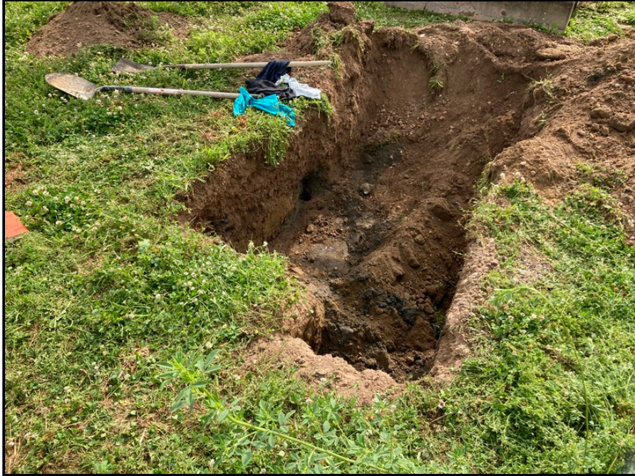
Excavation exposing the tops of AOCs 1D and 1E
